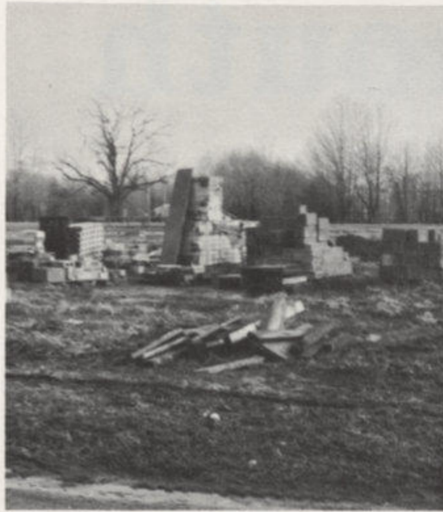
Bricks, blocks, and lumber, the beginning of a new look.
