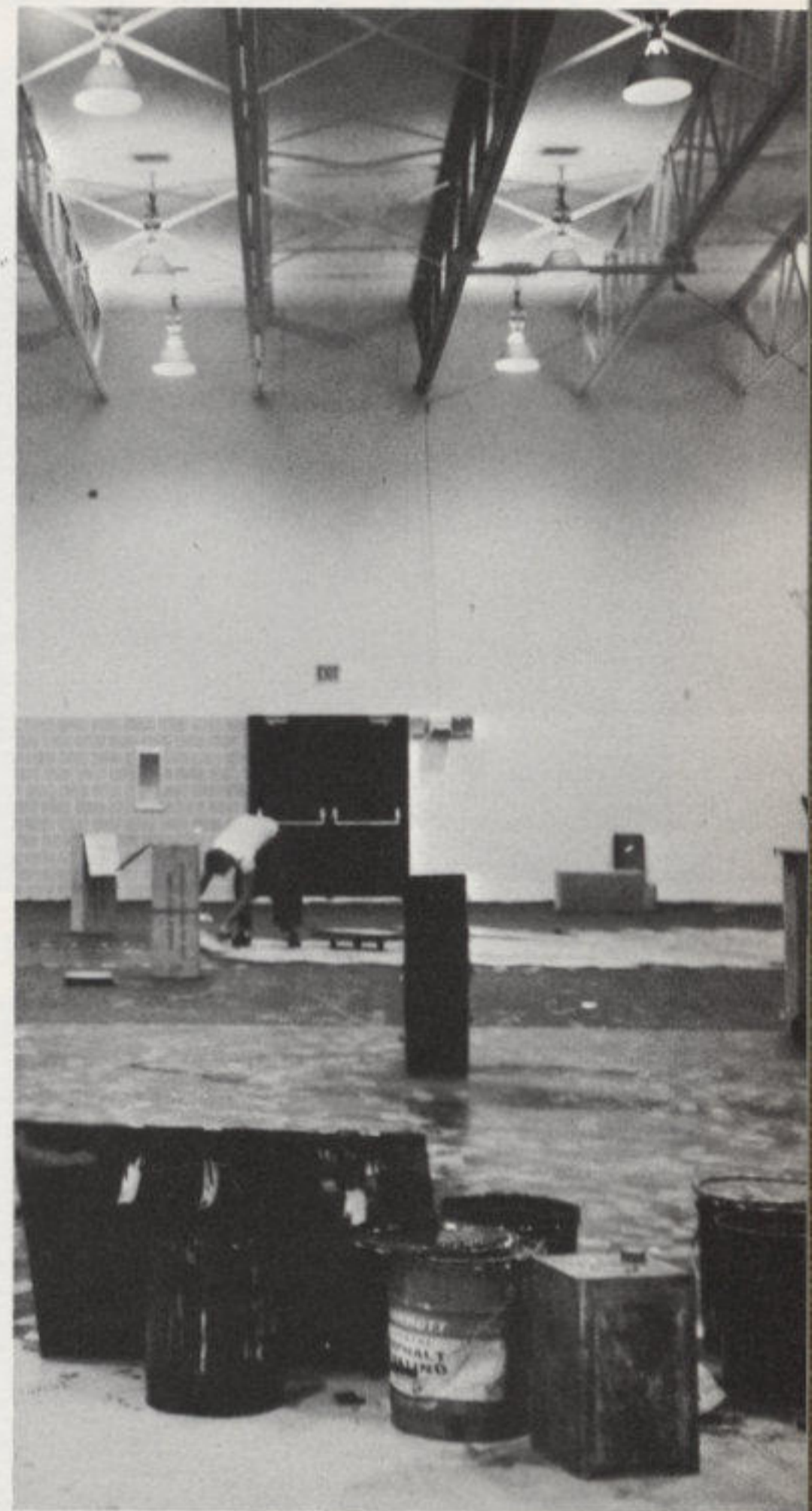
Gym floor is sealed and the wooden strips put in place.
