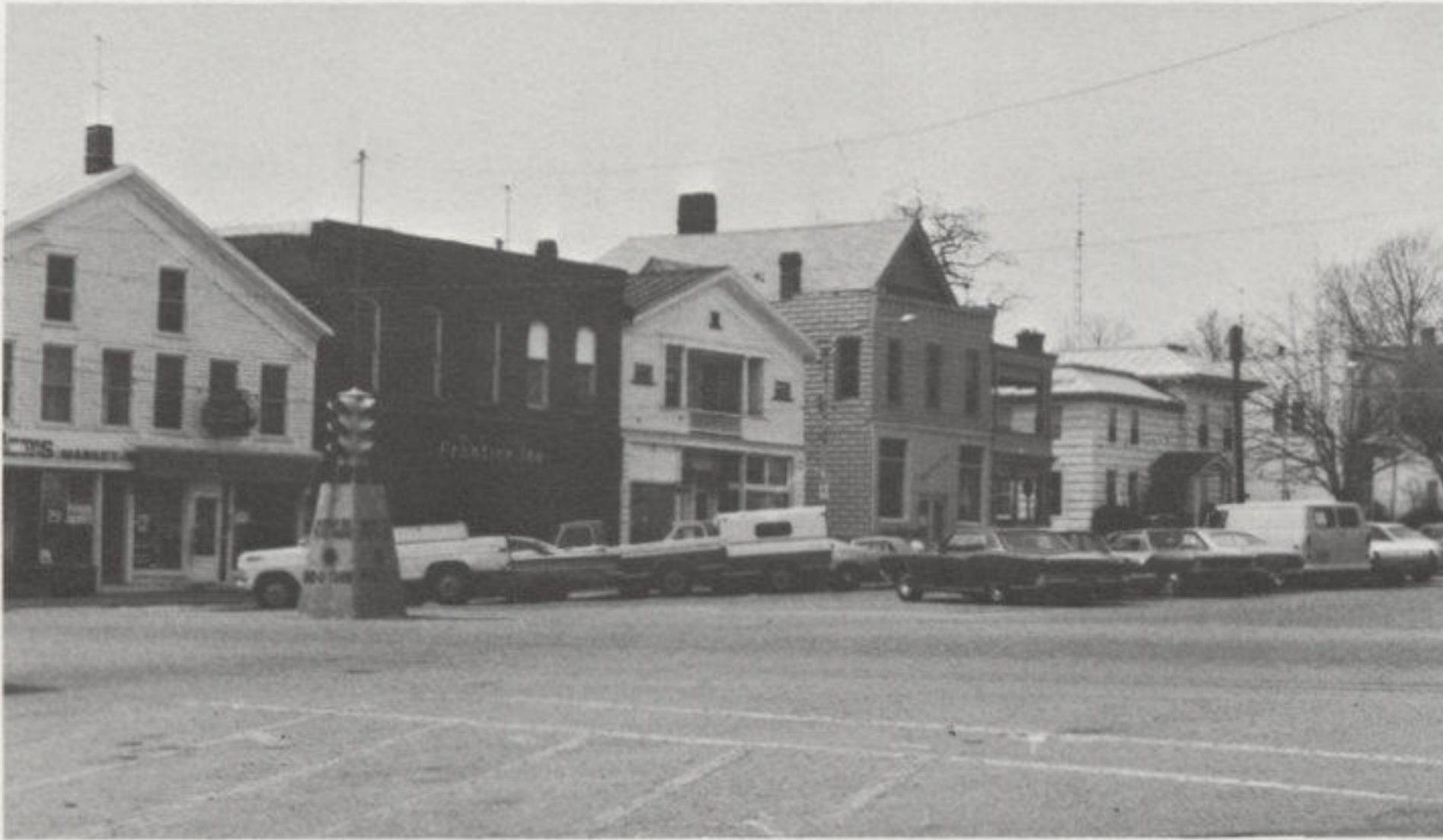
One of the last pictures taken before the dummy was removed.
