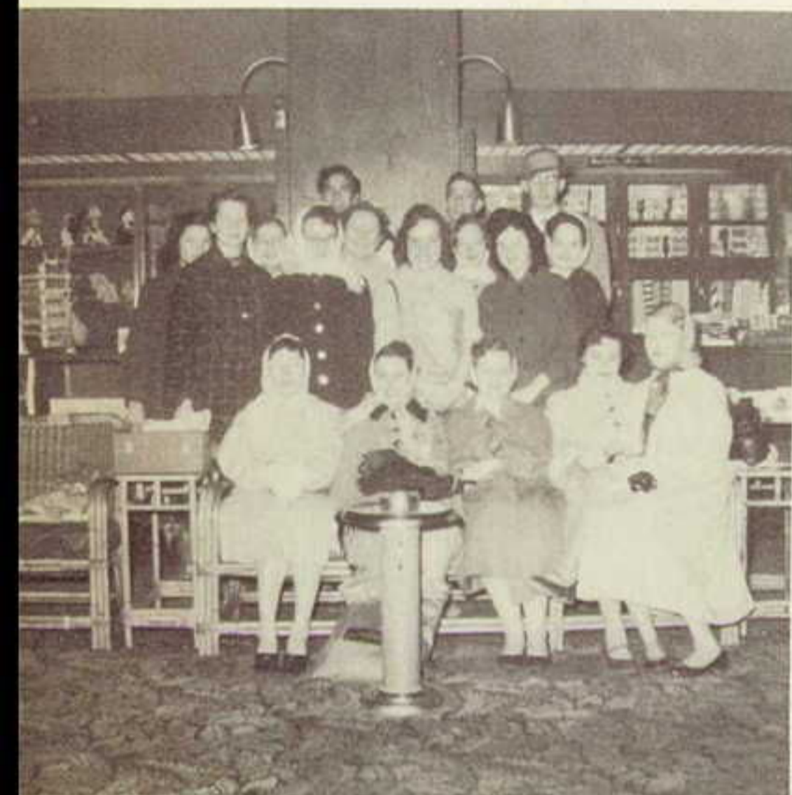
In Neil House Lobby in Columbus
