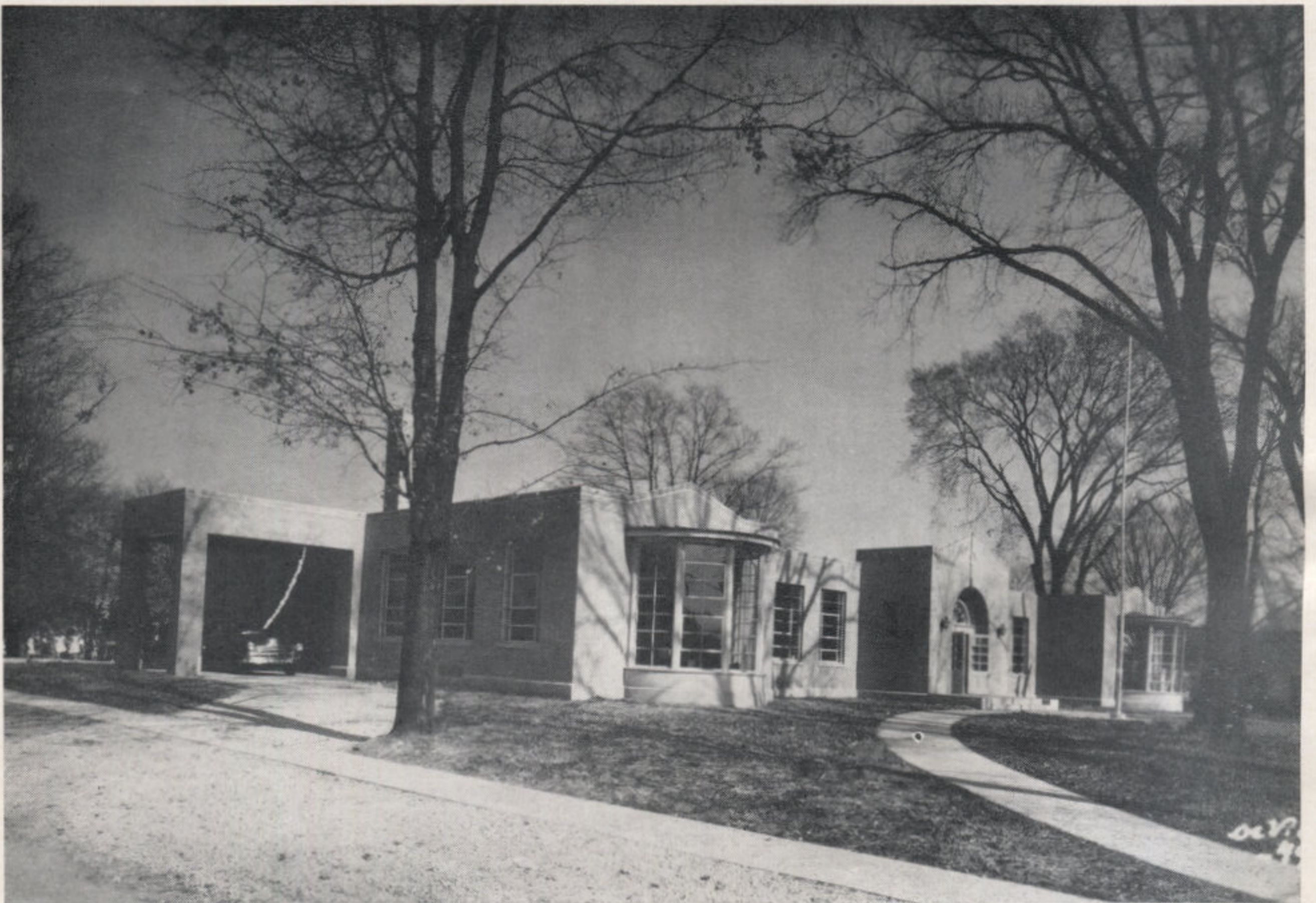
THE ELEMENTARY SCHOOL
